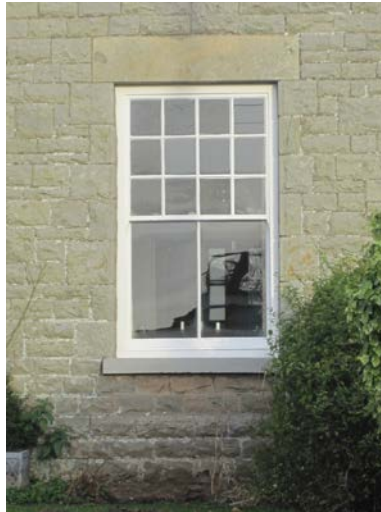
Sandstone plinth and quoin around window
