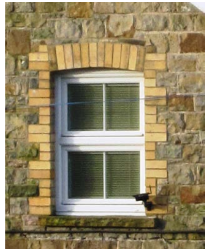
Brick quoin detailing around window
