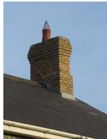
Pitched roof with chimney on ridge line
